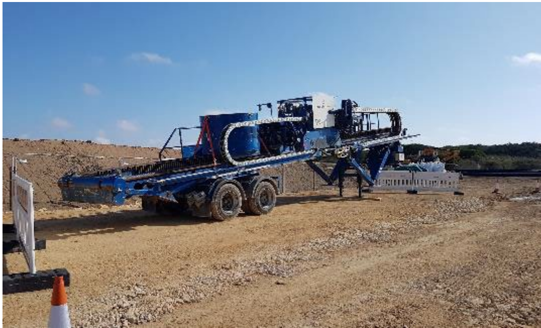
Plate 5.24 HDD rig (image courtesy of RWE Renewables)
