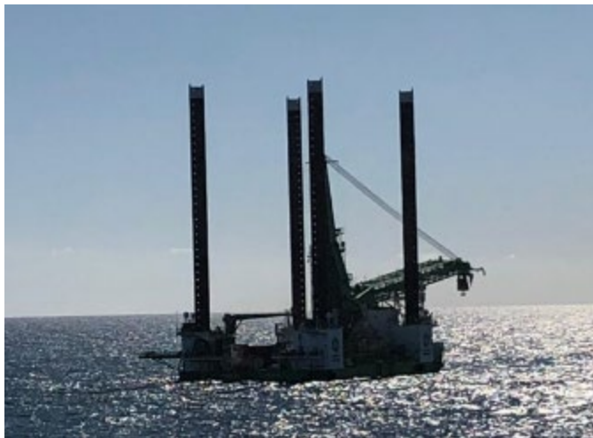
Plate 5.14 Example jack-up barge (image courtesy of RWE Renewables)
