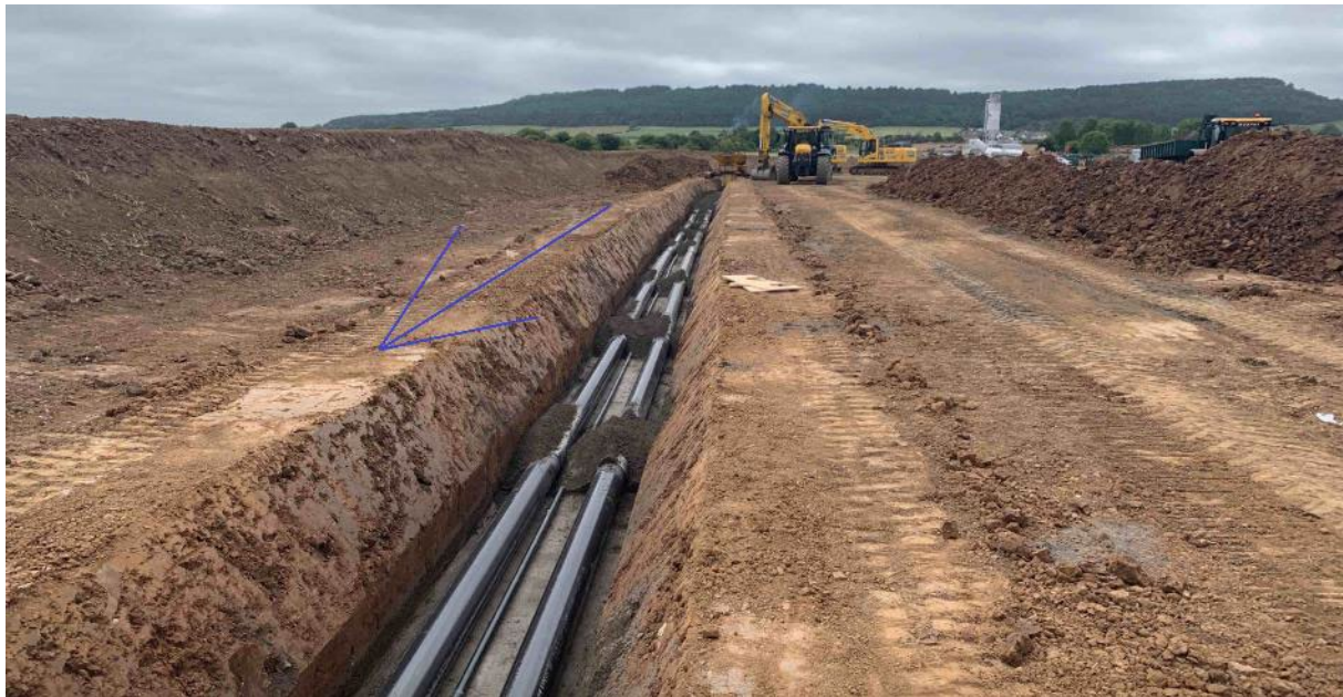
Plate 5.21 Typical open cut trench (image courtesy of RWE Renewables)
