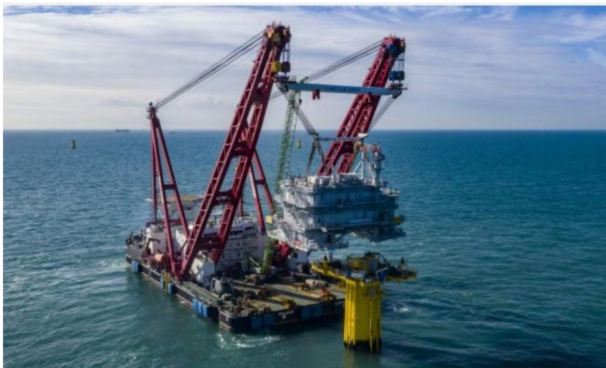
Plate 5.11 Indicative OSP topside installation (source: EnergyFacts, 2020)
