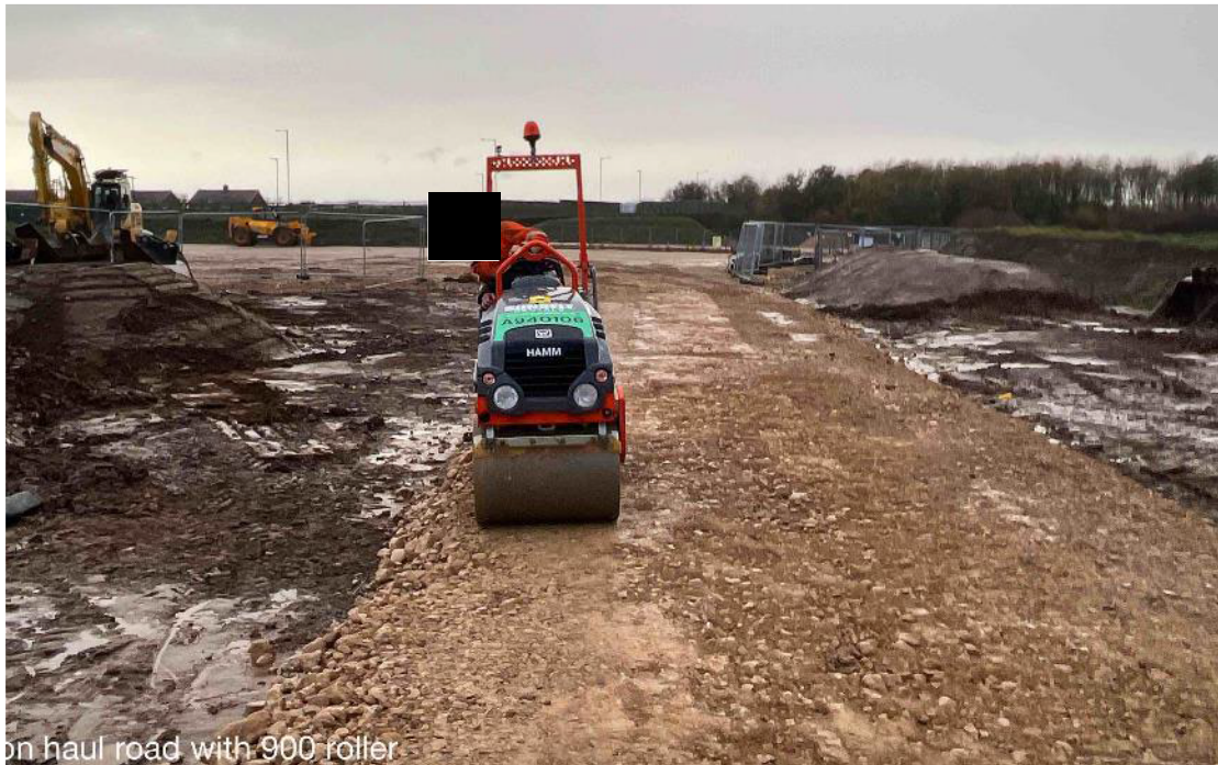
Plate 5.19 Example haul road (image courtesy of RWE Renewables)
