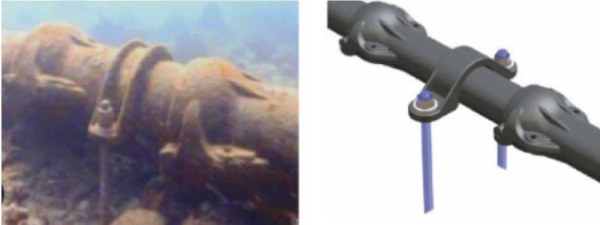
Plate 5.10 Indicative cable clip (source: Reda et al, 2021)
