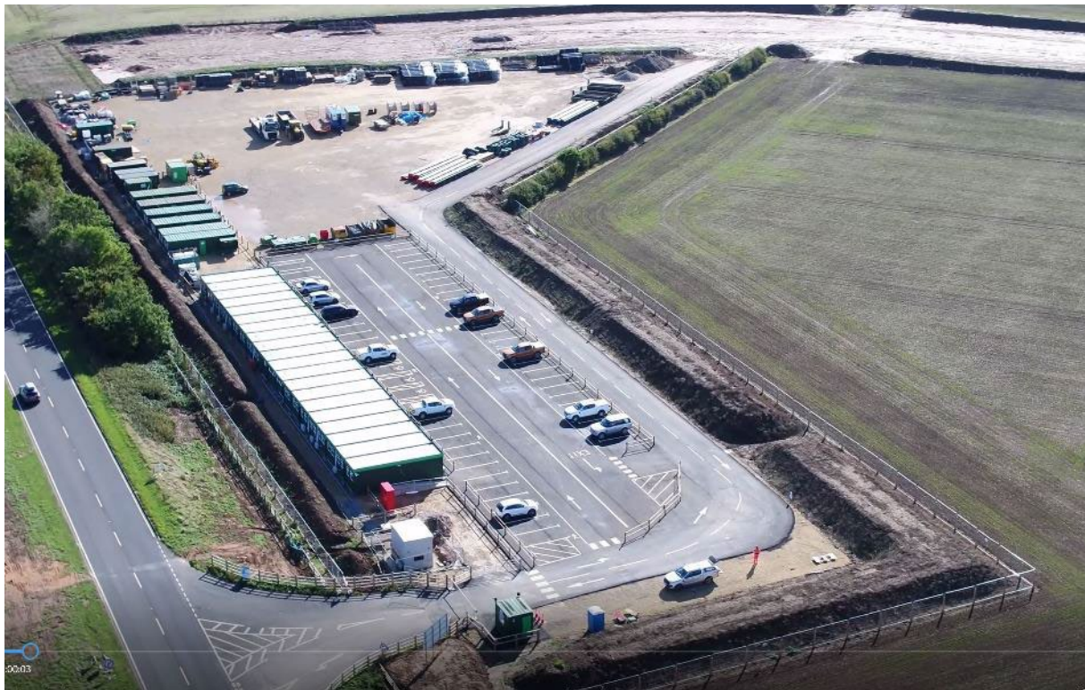
Plate 5.18 Example TCC (image courtesy of RWE Renewables)
