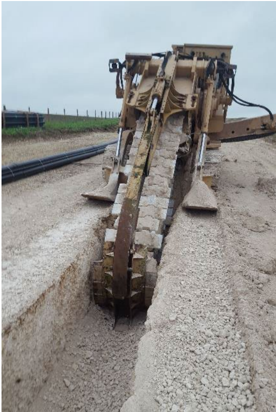
Plate 5.22 Example cable trenching machine (image courtesy of RWE Renewables)
