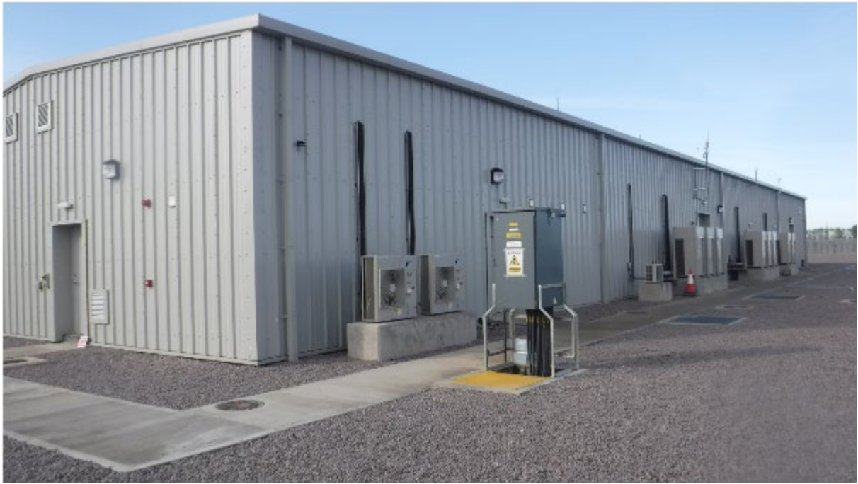
Plate 5.27 AIS control building (image courtesy of RWE Renewables)
