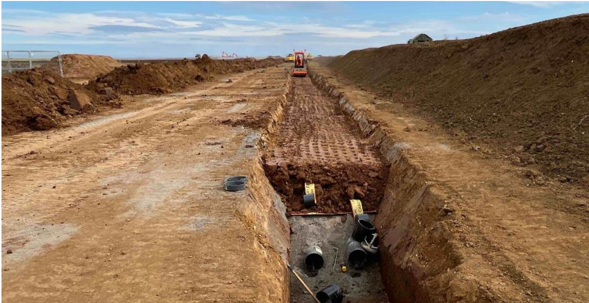
Plate 5.23 Example a backfilled trench (image courtesy of RWE Renewables)
